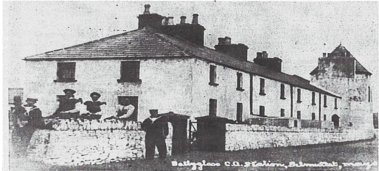
Ballyglass Coastguard Station. This building stood on the Western side of Broadhaven Bay and was occupied until 28th August, 1920, when the personnel were evacuated by a British destroyer. On the following day the station was burned by Republican forces to prevent it being re-occupied. Nothing of the building remains to-day. The original of this photo is in the possession of Mr. Jack Barrett, Knockshanbo.
